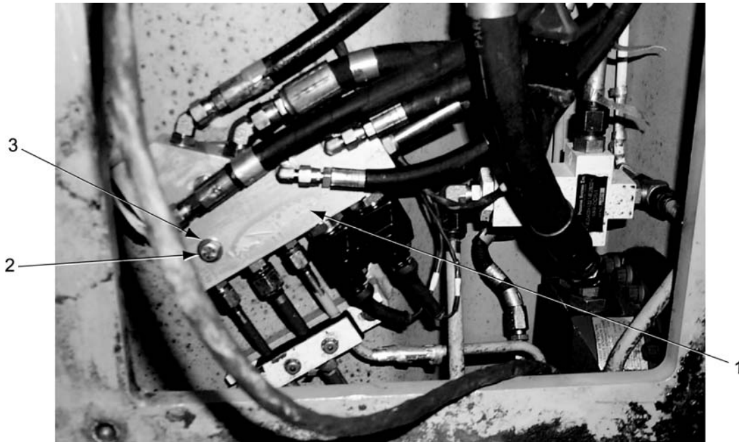
Figure 4-4. Installation of New Forward Left Manifold Assembly
